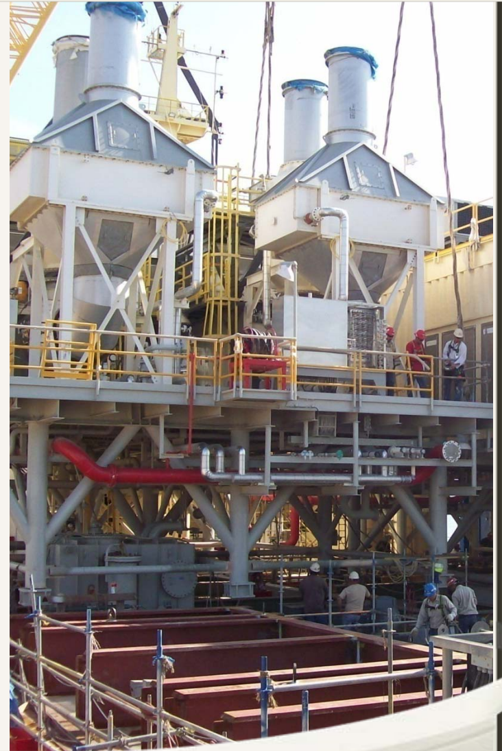
HPI production module installation
