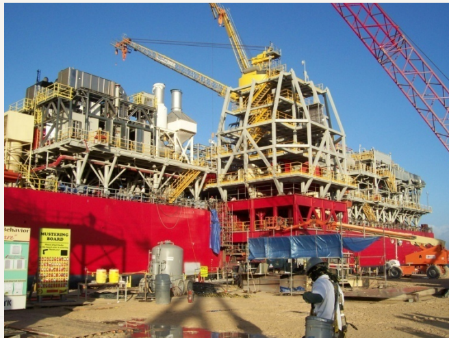
HPI external thruster porches, DTS receptacle and all production modules installed
