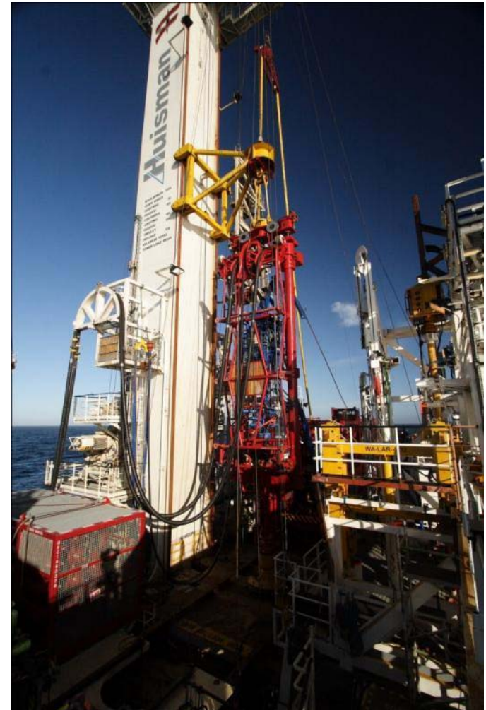
The Compensated Coiled Tubing Lift Frame on the Well Enhancer during its first coiled tubing operation
