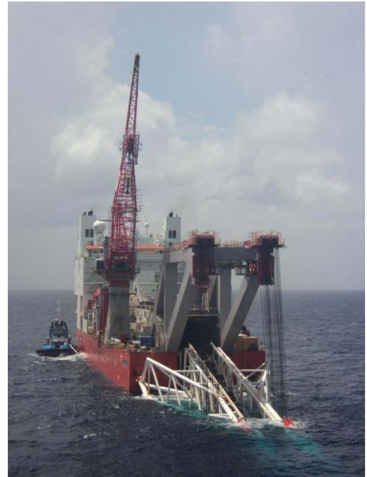
Caesar installing EOG Toucan pipeline offshore Trinidad
