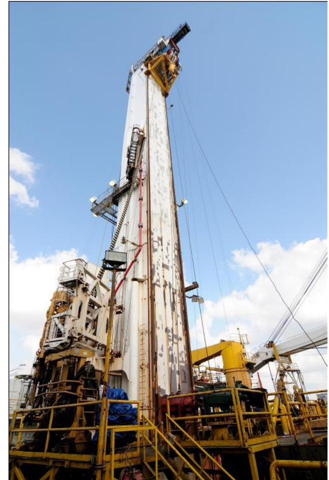
MODU DP3 Q4000 Multipurpose Tower undergoing paintwork at dry dock
