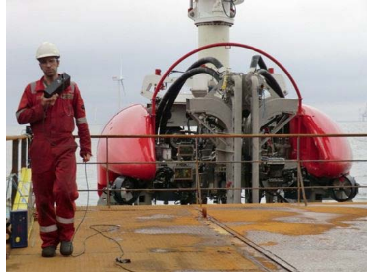
T1200 trencher being deployed
