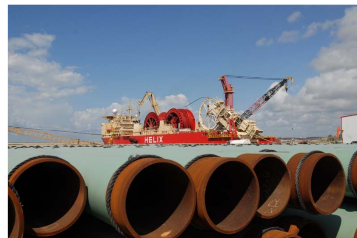
Express spooling pipe in Ingleside
