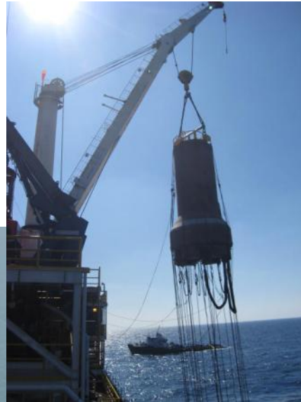
DTS Buoy being installed by Q4000
