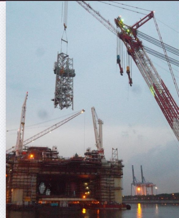
NOV tower being installed on the Q5000
