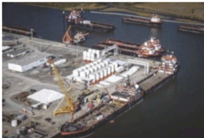
HOS Port Facility in Port Fourchon, Louisiana
