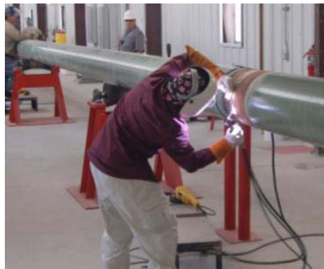
Helix Danny pipe welding
