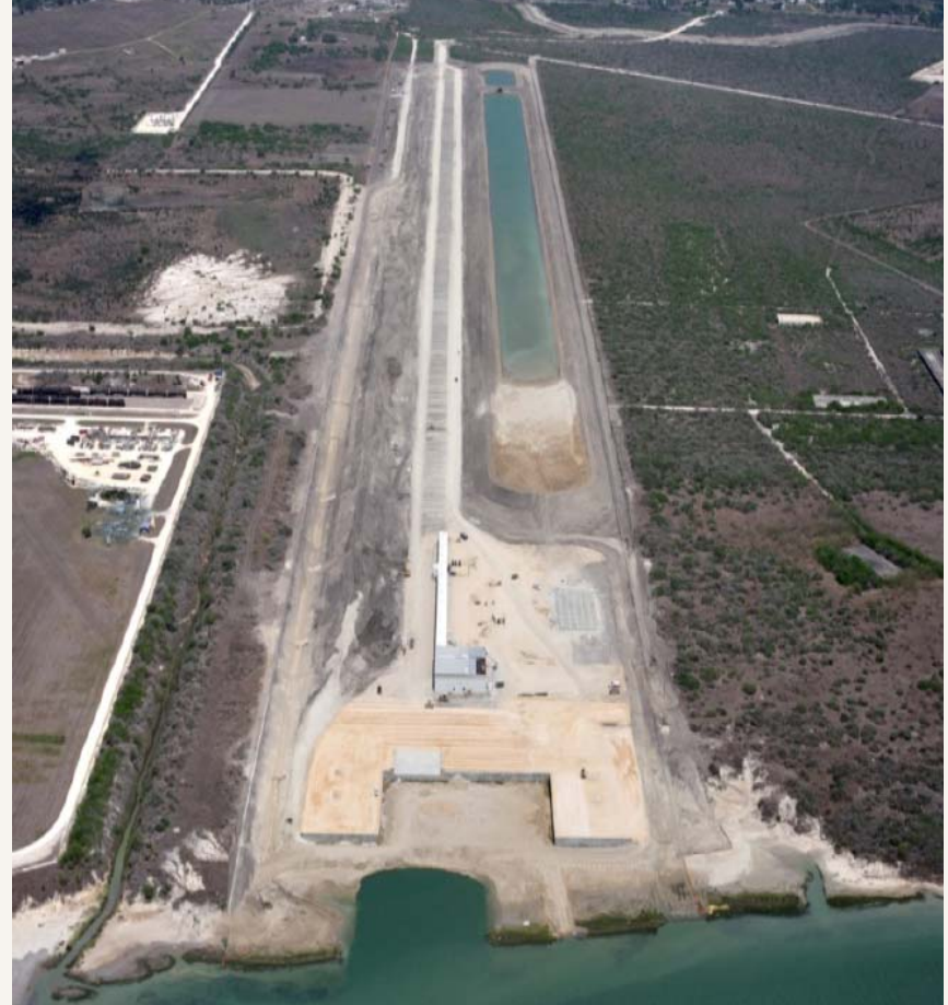
Aerial view of Ingleside Spoolbase, with slip dredging project underway
