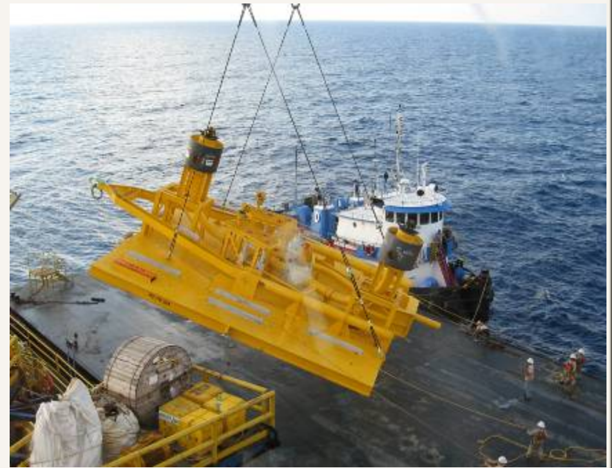
Murphy Thunder Hawk PLEM being lifted onto Intrepid from transport barge
