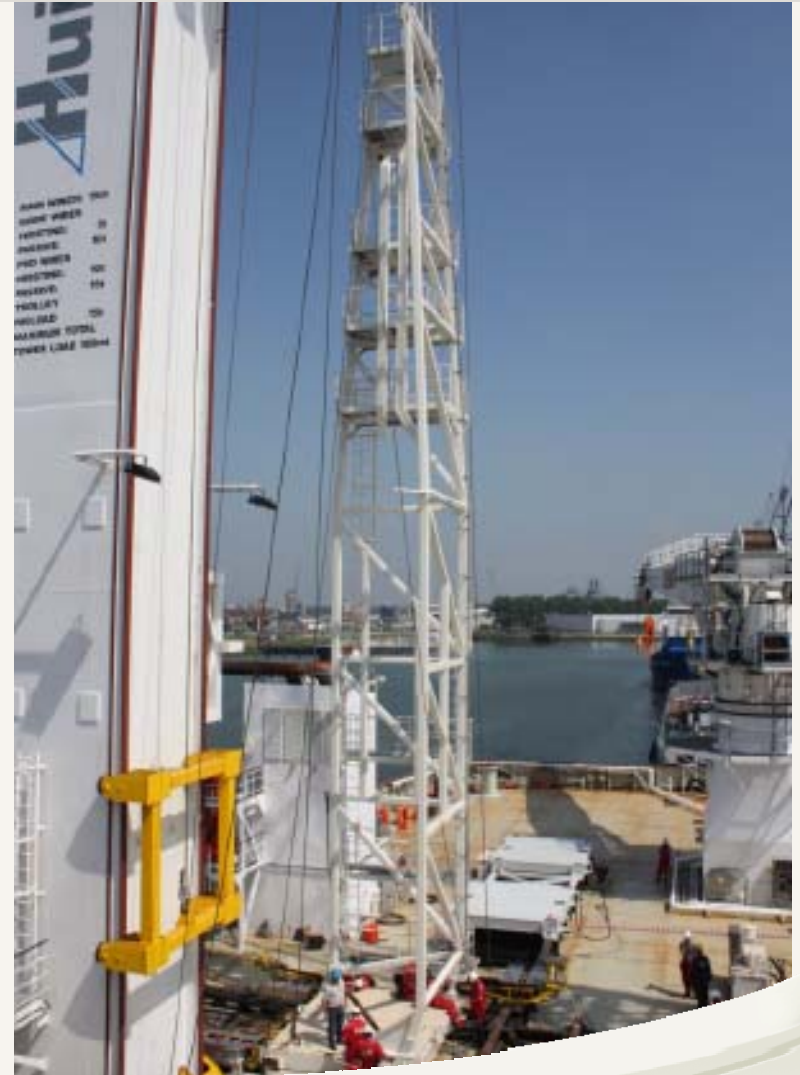
Subsea Intervention Lubricator access tower installed on Well Enhancer deck
