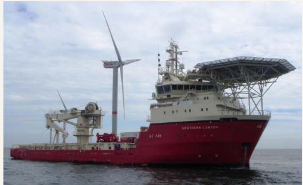
Northern Canyon burying power cables for North Sea wind farm
