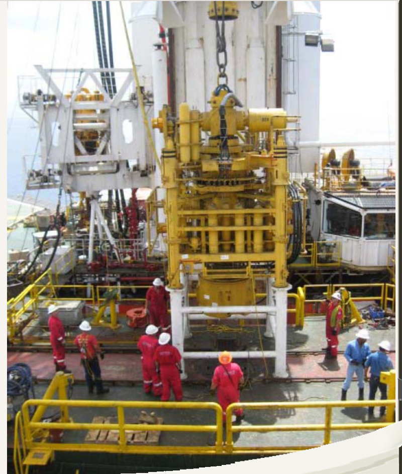
Subsea Intervention Lubricator system on board Q4000
