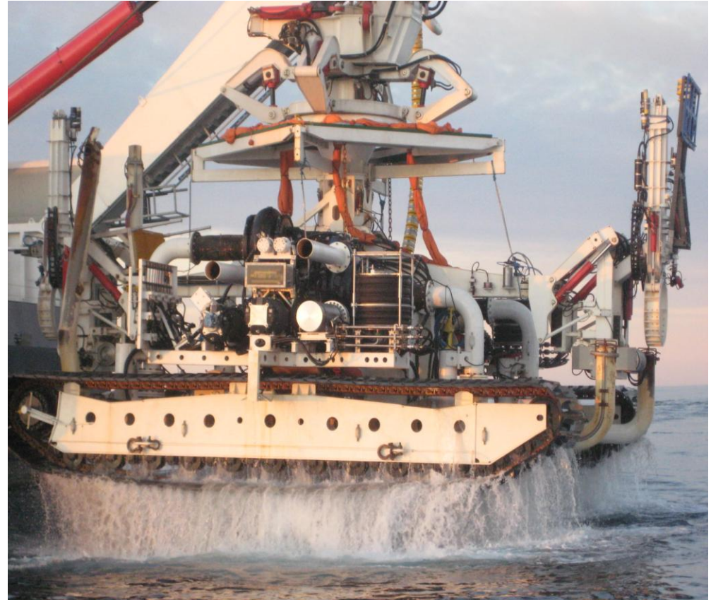
iTrencher being deployed off of the Island Pioneer in the North Sea
