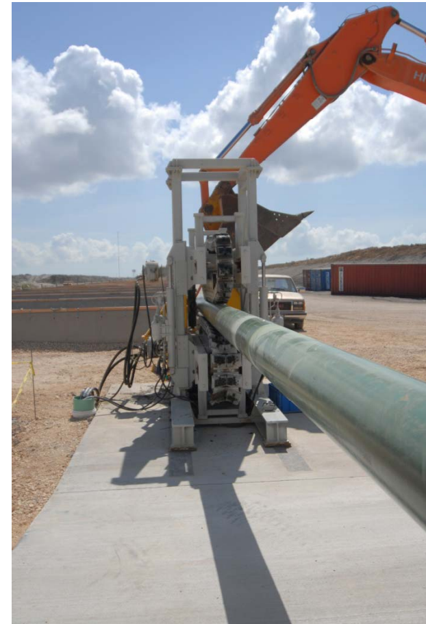
Welding and spooling pipe at Ingleside Spoolbase
