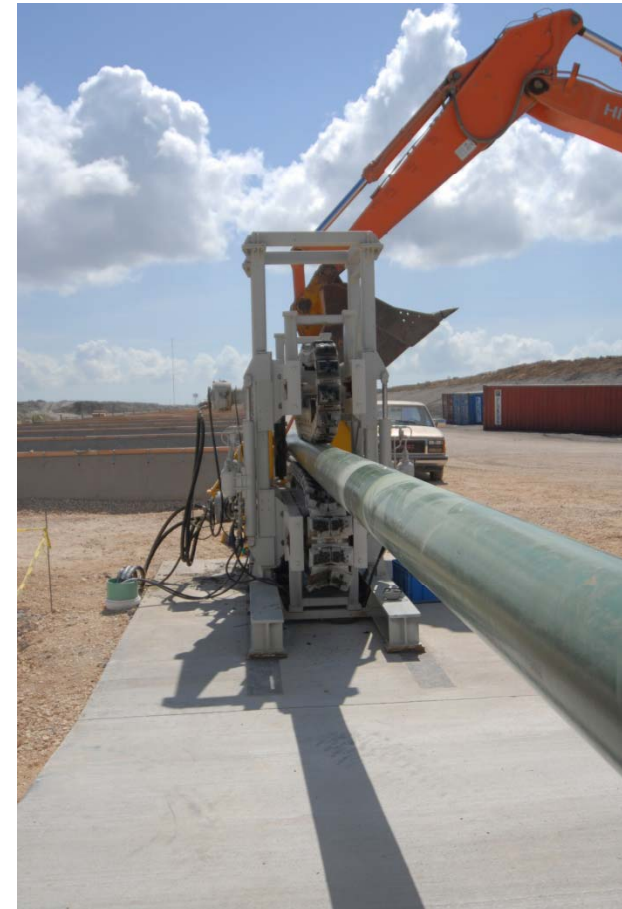
Welding and spooling pipe at Ingleside Spoolbase
