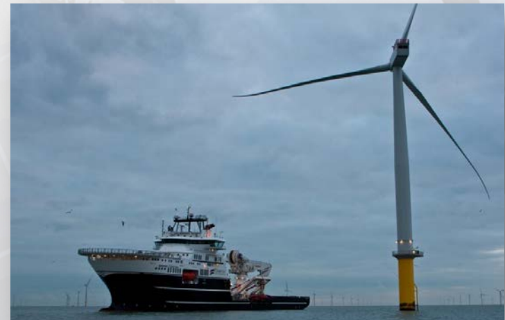
Grand Canyon deploying the T1200 Jet Trencher
