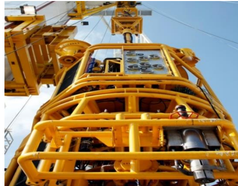
Intervention Riser Systems 1
